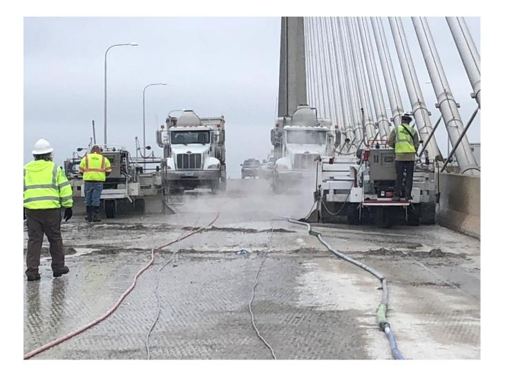
The work includes a combination of surface milling and 3/4" Fast Track Hydrodemolition to prepare the deck surface for a new 1-3/4" concrete inlay. The total surface area of hydrodemolition and concrete inlay is 137,000 square yards. Hydro-Technologies, Inc. is utilizing two hydrodemolition robots in order to minimize the work shifts on the tightly scheduled project.
