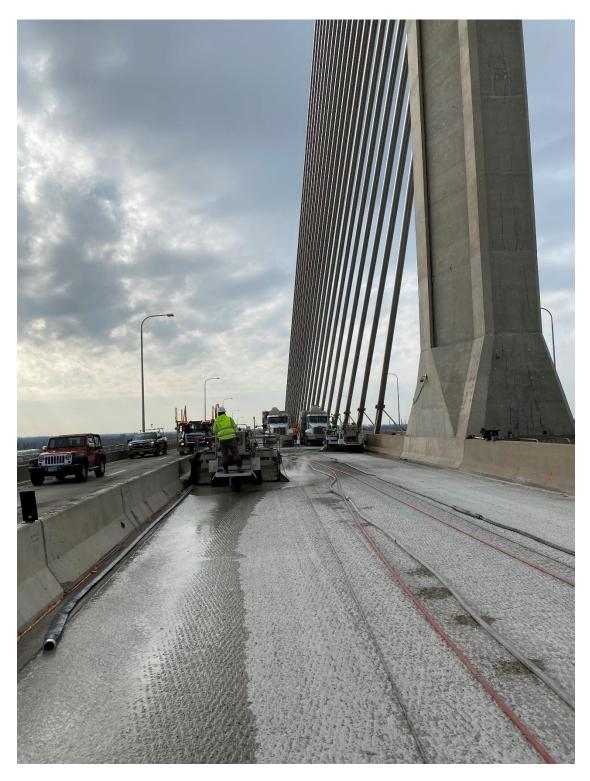
One of the unique aspects of this job is the care needed to insure the post-tensioning ducts in the bridge deck are not damaged during the concrete removal and preparation process. That makes the Fast Track method of hydrodemolition very well-suited for this project. Hydrodemolition also does the work dust free and in an environmentally friendly manner.
